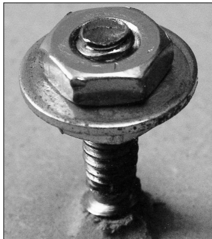
PHOTO 31: Mounting a hanger bolt.
