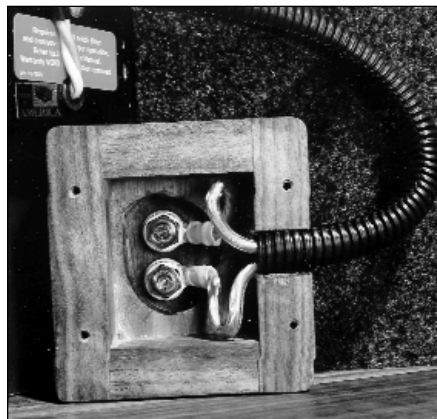
PHOTO 32: Attaching speaker leads.
