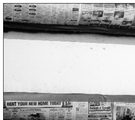
PHOTO 22: Masking before painting.
