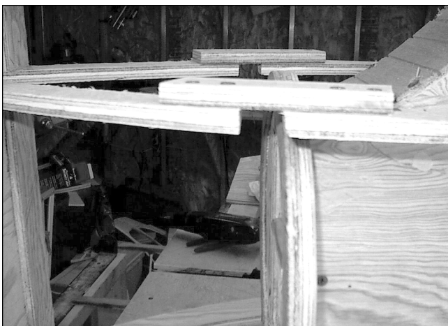
PHOTO 14: Horn braces cut in two pieces with stabilizing cauls attached.
