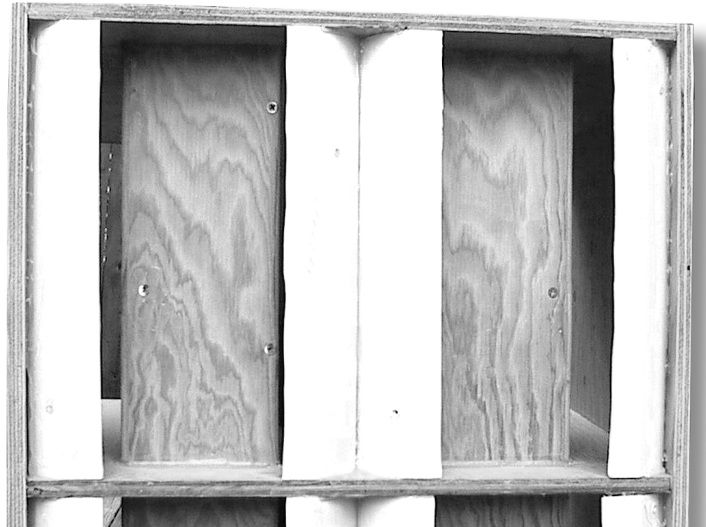
PHOTO 19: PVC throat reflector installation.
