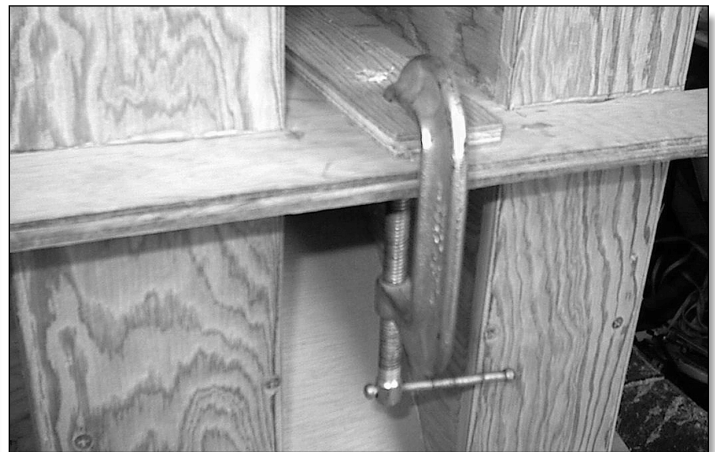
PHOTO 16: Installing the back brace.
