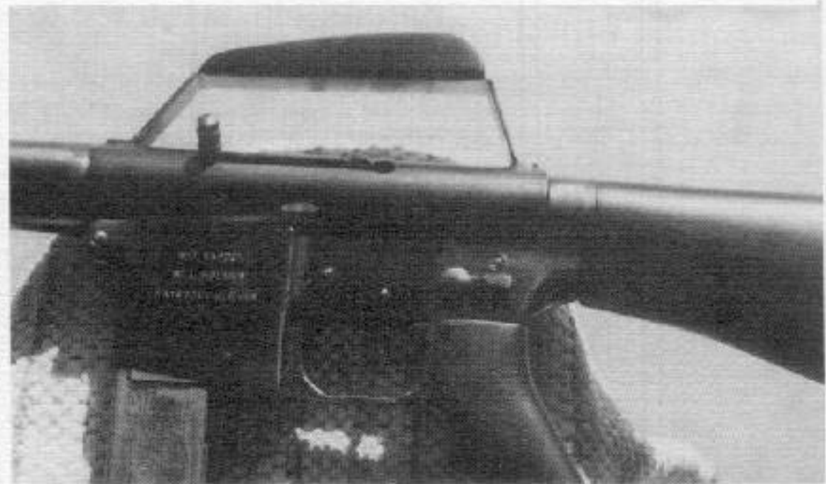
Finished rear sight mounted in place.
