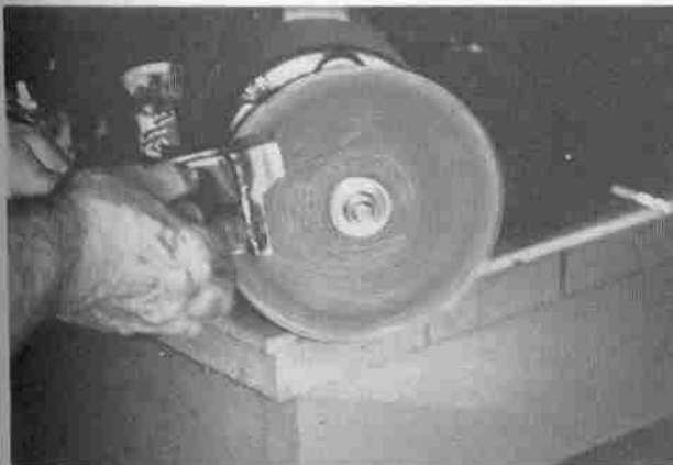
Welds are ground flush with disk sander.
