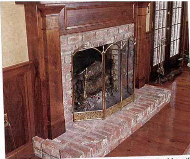
Erickson built this mantel for a fireplace on a raised hearth. The fireplace mantel extends away from the wall approximately 4 in. to accommodate the fireplace's facing bricks, which were laid proud of the wall.
