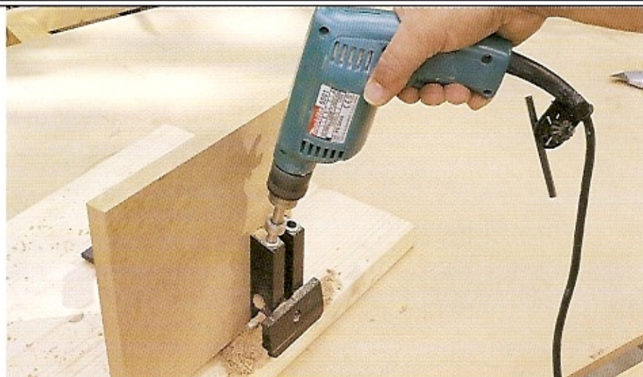
8 Drill pocket holes in the shelves.
