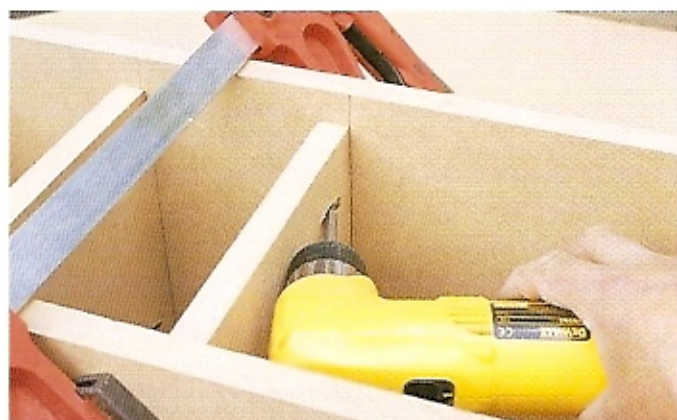
10 Attach the other tower side to the shelves using pocket-hole screws.
