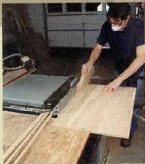
CUT THE SLATS. After applying backing veneer to one side, rip the panel into slats. A double-width push stick and a slow, steady feed rate help keep the slat tight against the fence.
