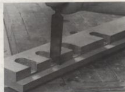
5/ Then clean up the edges of the notch with a chisel.
