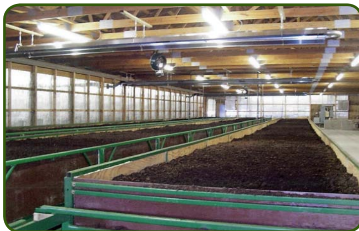
Figure 2.3 A large-scale vermicompost facility with raised beds to hold organic materials that are broken down by earthworms. Finished vermicompost is on the bottom of the beds and drops into some type of receptacle underneath the beds.
