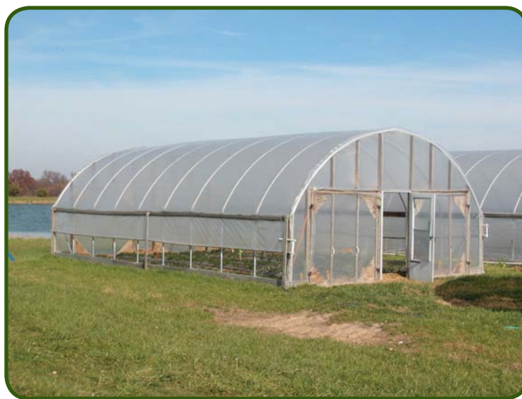
Figure 11.4 A high tunnel structure near Columbia, Missouri.
